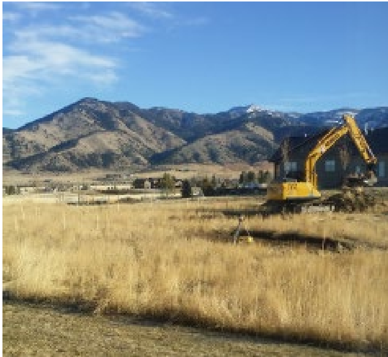
Studers’ jobsite – November 30 (Doc. 4, Am. Compl. at 16).
